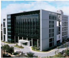
Taoyuan Technology Center (Green Building)
