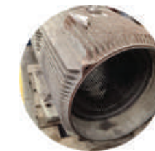
Annealing of electric machine winding insulation
